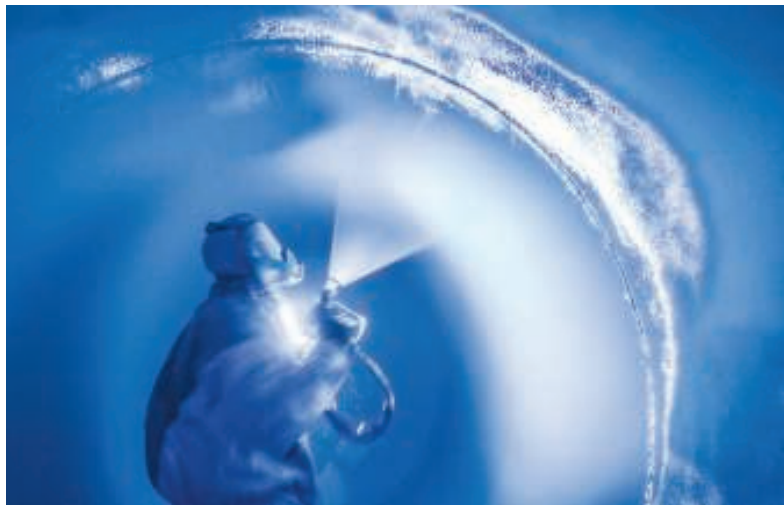
FIGURE 2. Series 391 Tank Armor from Tnemec is a chemical-resistant formulation for use in severe chemical-immersion environments
